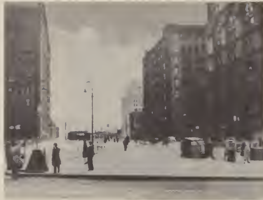
Entrance to the Bridge from the Manhattan end, prior to reconstruction, with trolley turnaround in background.
